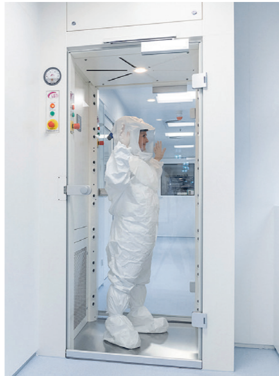
The air shower provides a safe working environment when handling highly potent substances.
